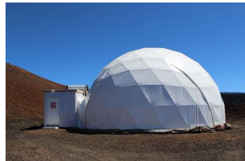
Figure 1. HI-SEAS habitat with doorway to airlock chamber
